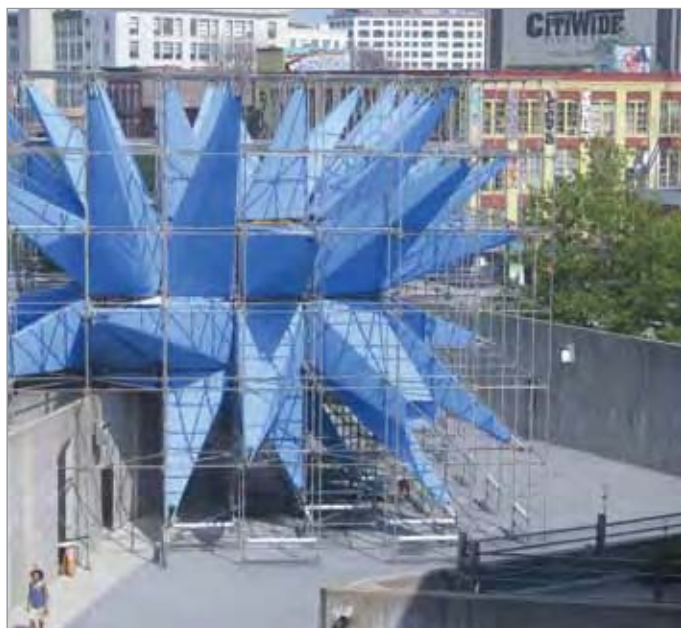
Figure 2. 'Wendy,' the winning design of MoMA's Young Architects Program in 2012. TiO 2 nanoparticles sprayed on its surfaces neutralize nitrogen dioxide air pollution.
